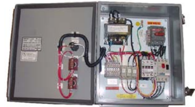
Custom built Starter shown above
